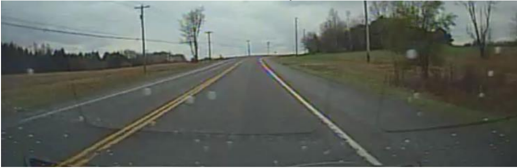
Moderate roadway furniture
