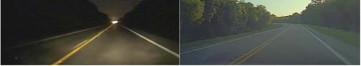
Pavement markings indicated as “highly visible”
