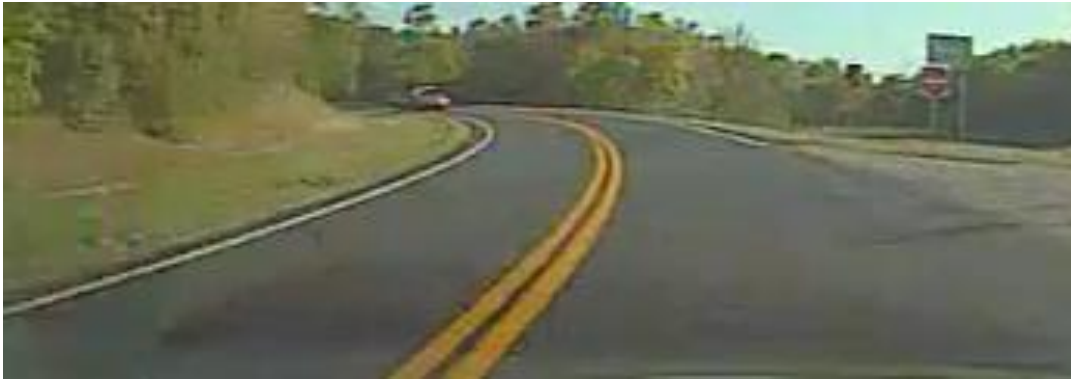
Pavement condition indicated as “normal”
