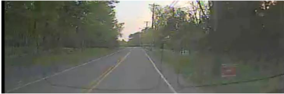
Large amount of roadway furniture
