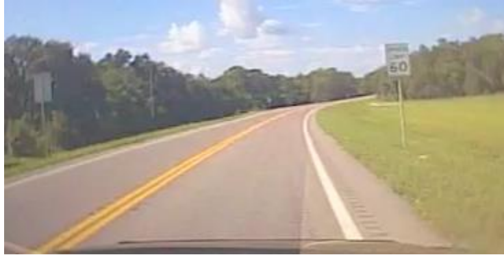
Figure A.3 Presence of edge line only rumble strips (image source: DAS forward imagery)
